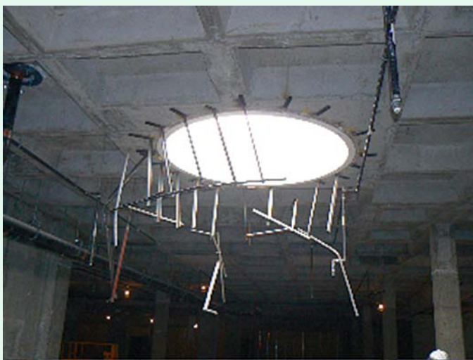
This skylight is where the old McHenry Library's signature spiral staircase was located. Though loved by many it was a fire hazard and had to go.
